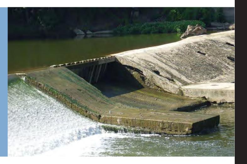
In 2010, the City of Frankenmuth decided to replace the aging structure with a new rock ramp or constructed rapids. The rock ramp opens up 73 miles of river and creeks, allowing fish to swim upstream to spawn. This is extremely important for the Saginaw Bay, enabling natural fish reproduction for the popular Walleye fishery. The rock ramp also allows the Cass River to keep the river profile needed to enable commercial and recreational boating.
